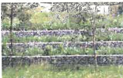
Murets gabions, photo DDF
