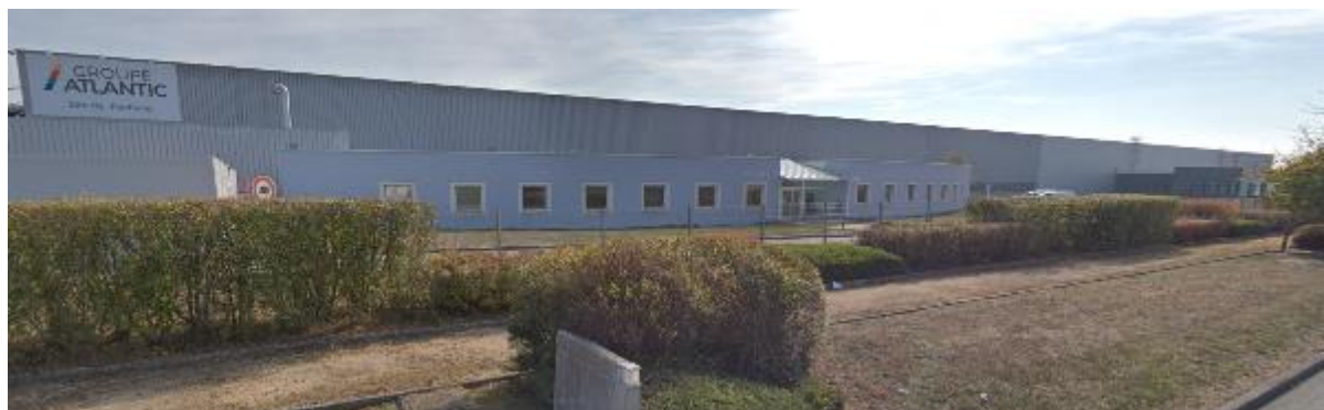
Installation 6 : ADLER France
